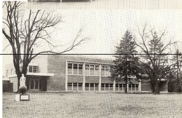
Weidler Hall Cafeteria and Student Union
